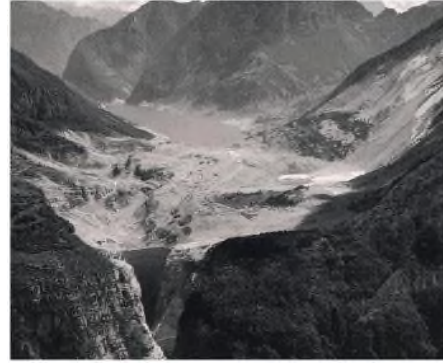
Figure 12.2 | An image of the Vajont reservoir shortly after the massive landslide (you can see the scar from the landslide on the right, and the dam is located in the foreground on the left).
