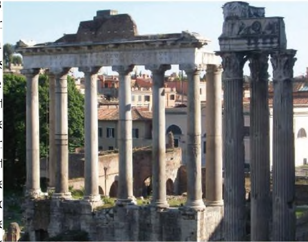
Figure 12.3 | This is a picture of the Roman Forum. Why did the Romans use so many vertical columns to hold up the one horizontal beam? If the horizontal beam spanned a long distance without support, it would buckle under its own weight. This beam is under tensional stress, so it is not as strong.
